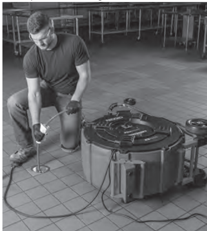
Figure 11 – Lubrification de la gaine de câble
