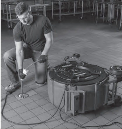
Figure 11 – Applying Lubricant to the Cable Sheath
